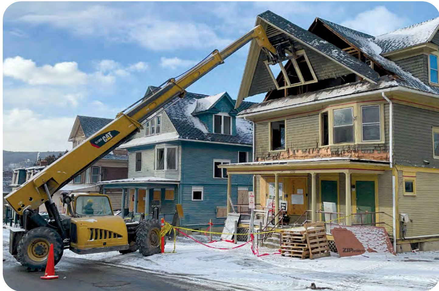
Deconstruction in progress, courtesy of Felix Heisel
